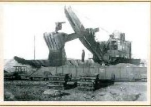
Menck & Hambroek electric shovel loading rail carriages
