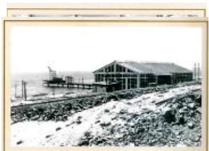
Lower station and jetty
