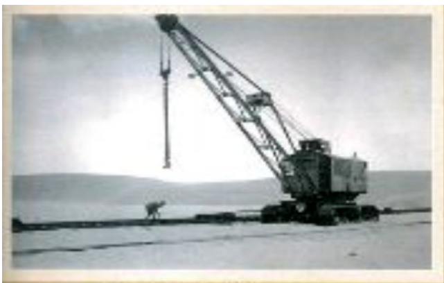
Laying the railway line
