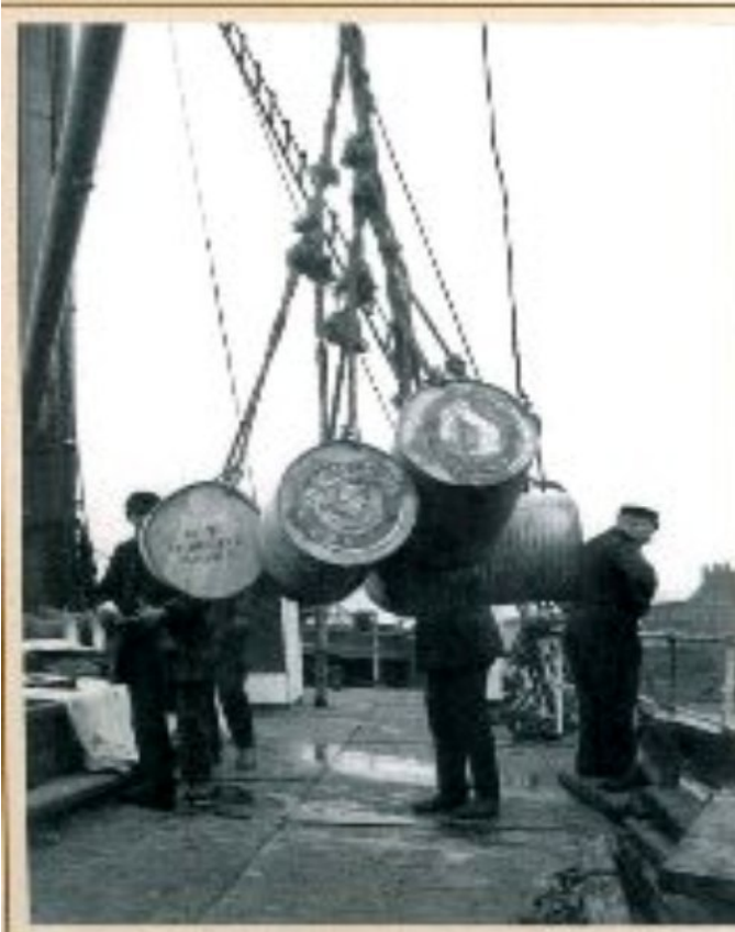
Unloading the German cement for Elizabeth Bay
